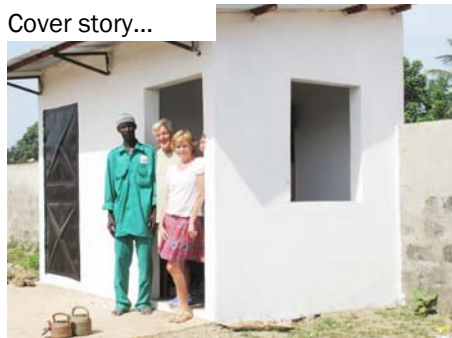
The new Watchman's hut and store room
